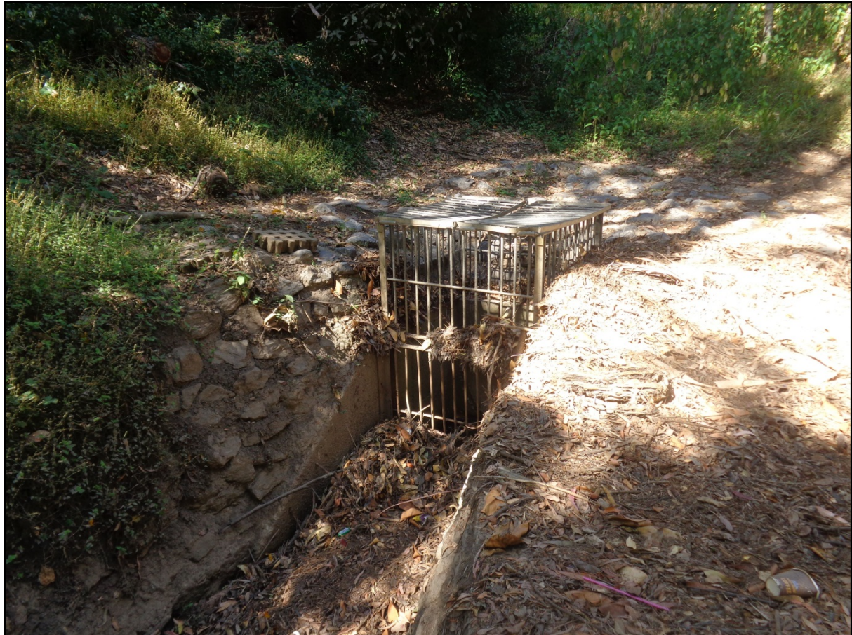
Figure 4.2: Detention Basin Low-flow Grated Inlet
